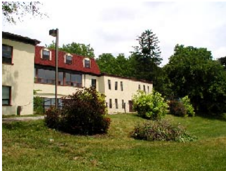
Cedarvale Park, view of some of the on-site buildings
