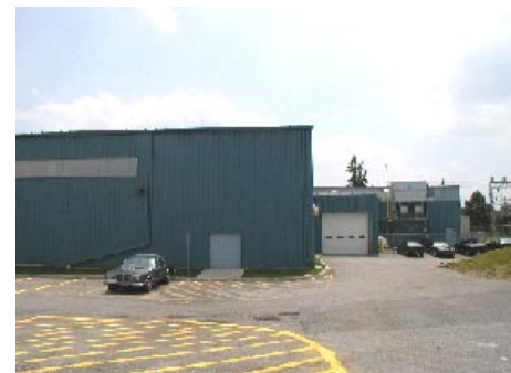
Proposed Library site behind Mold Masters Sports Complex Arena
